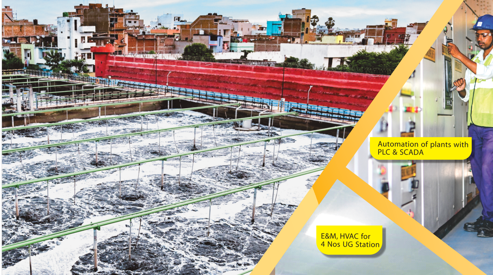
Pumping Station & STP-Patna, Bihar
