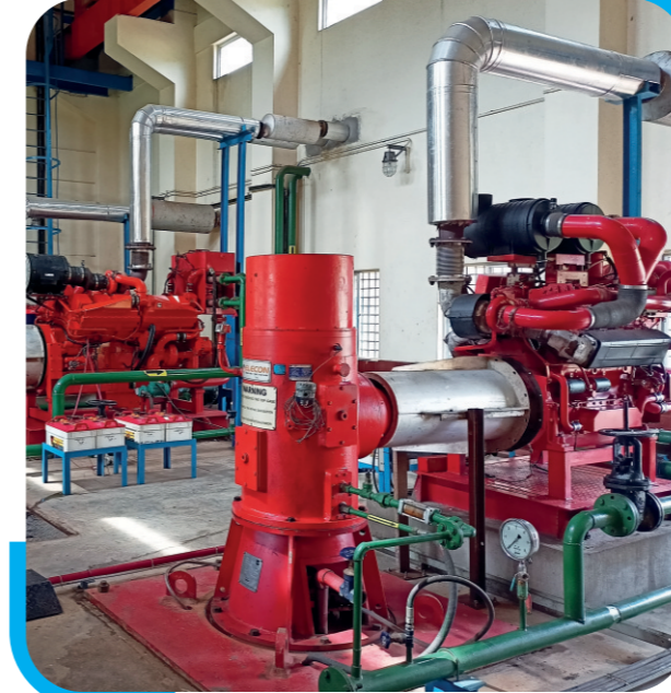
OWSSB- Diesel generator based Storm Water Pumping station
