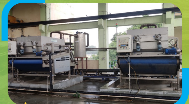
★ UPJN- Agra - WTP Belt Filter Press
